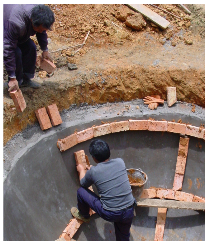
Construction of a biogas digester—ID
