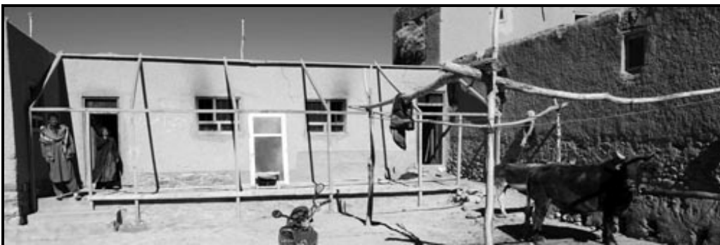
Picture 10: Installation of PSH before the winter
