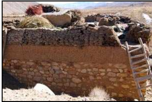
Picture 5: the roof, storage of bushes and dung
