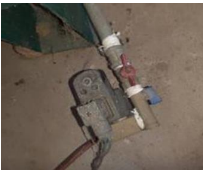
Example of audit drain valve
