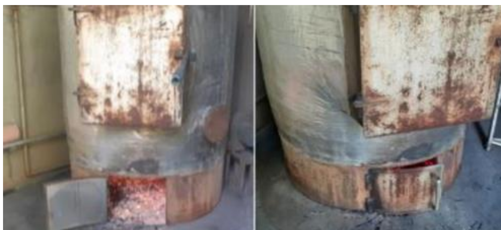
Present door position and suggested door position
