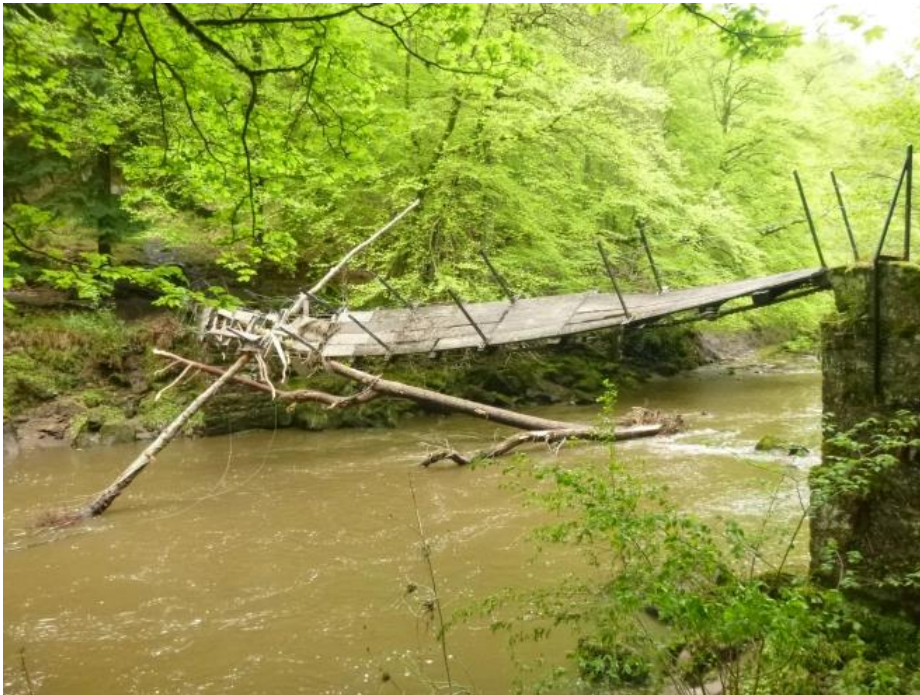
Visual 3: Almost dysfunctional/collapsed bridge
